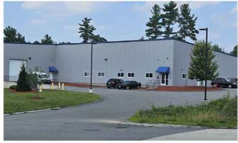
Hudson, New Hampshire (Under Construction)
